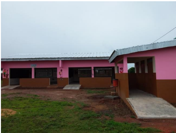
Notes: Community preschool, with both classrooms (back), the sanitary facilities and the handwashing station (right)
